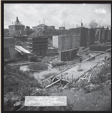
ST. MARYS RIVER, MICHIGAN 4TH LOCK MASONRY UNLOADING TRUSSES FOR FORMS LOWER GATE RECEIVED JANUARY 31 1917
